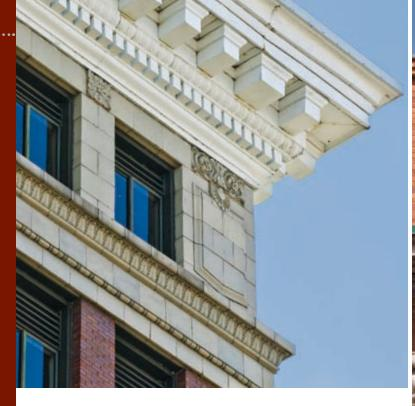
The weight of the building is handled by a steel frame instead of the masonry walls, an important innovation at the time that enabled skyscrapers to become a reality. Chicago architect Jenney is now recognized as the "father of the skyscraper." The Jefferson Building was billed as "Peoria's first fire-proof building." WHERE: 331 FULTON STREET BUILT: 1910 Architect: William LeBaron Jenney Style: Classical Greek Revivial
